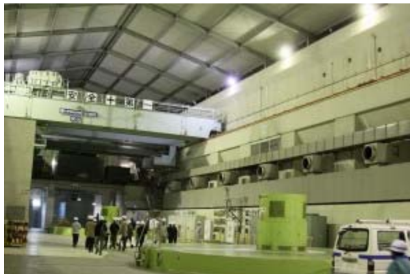
The large hall housing the Tenzan underground hydraulic power plant in the Sefuri mountains
