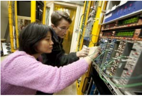
Two participants in a hands-on training session inspect the electronics for their test beam measurement at Fermilab this month. Photo: Fermilab
