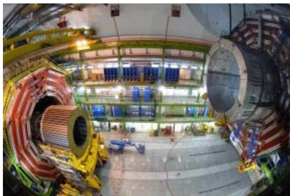
Lowering of the CMS parts into the experimental cavern. The ILC detectors are of similar size. Image: CERN
