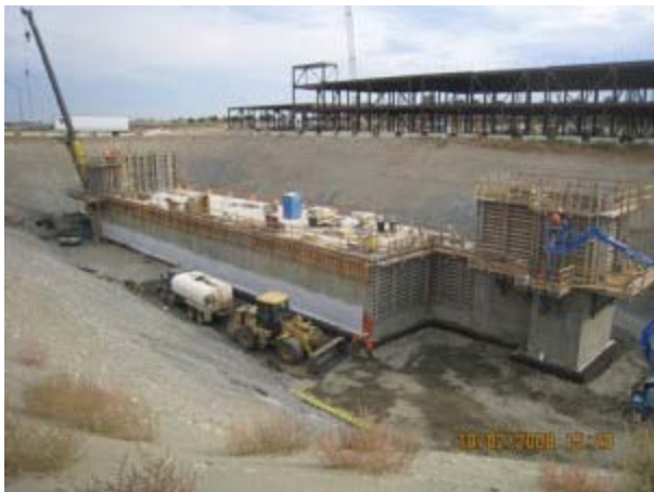
A shallow underground laboratory at the DOE Pacific Northwest National Laboratory at Hanford.
