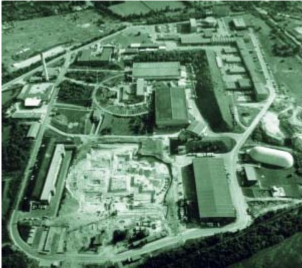
The DORIS construction site in 1970. Image: DESY
