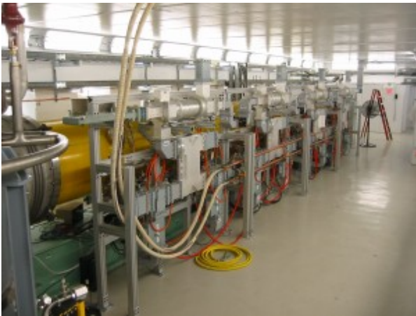
SLAC-developed waveguide system installed with a Fermilab cryomodule. Photo: Jerry Leibfritz
