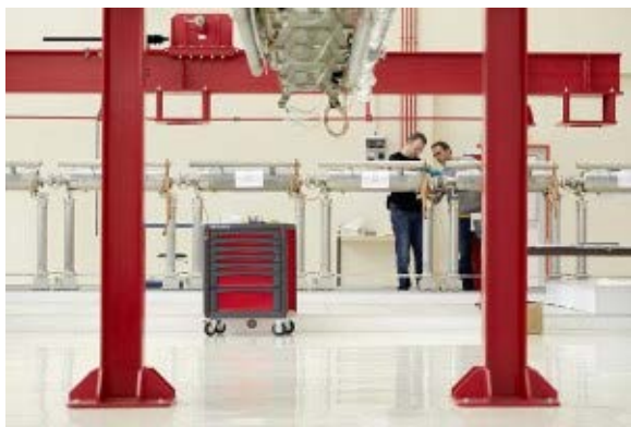
Cryomodule assembly at CEA, Saclay, France. (Image: DESY/ILC, photographer: Heiner Müller-Elsner)
