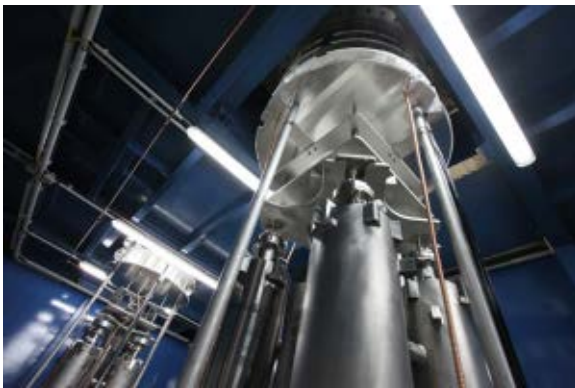
Vertical test inserts equipped with XFEL superconducting accelerator series cavities. Image: DESY
