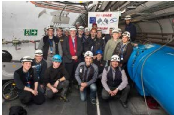
Consolidation works in the LHC tunnel during LS1 are nearing their end. Image: CERN
