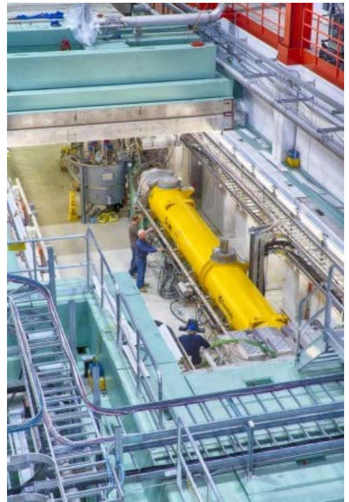
CM2 in its home at Fermilab's NML building, as part of the future Advanced Superconducting Test Accelerator. Photo: Reidar Hahn
