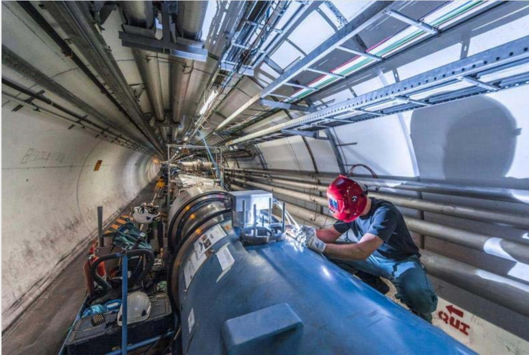
A welder at work consolidating interconnections between dipole magnets on the Large Hadron Collider (Image: CERN)
