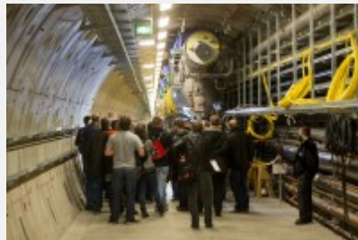
Inside the tunnel of the European XFEL.
