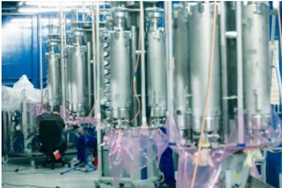
In the preparation area, six vessels can be equipped with four cavities each. Images: Dirk Nölle, DESY
