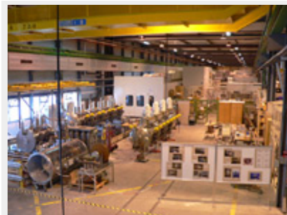
'SM18' at CERN: This is where the proposed test facility could be installed when LHC tests are finished.
