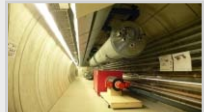
Almost like the real thing: the mock-up tunnel for the European XFEL. By the way, the klystron and transformer are made of wood. Photo: DESY
