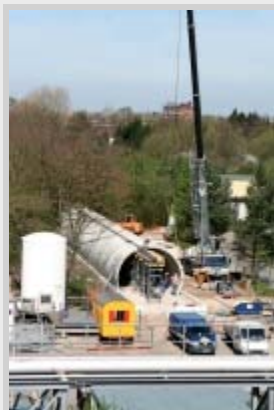
DESY has built a tunnel above ground to test XFEL linac installations. Photo: DESY
