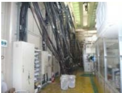
The primary damage to ATF, with fallen cable racks and cables. It will require about a month to repair. Image: Nobuhiro Terunuma
