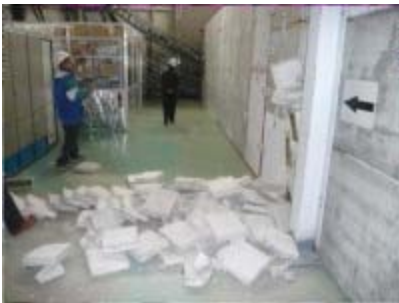
Fallen ATF2 shield blocks. Image: Nobuhiro Terunuma
