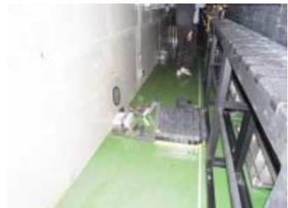
Fallen and overturned lead blocks at KEK's linear accelerator. Image: Nobuhiro
