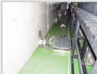
Fallen and overturned lead blocks at KEK's linear accelerator.
