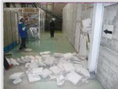
Fallen ATF2 shield blocks.
