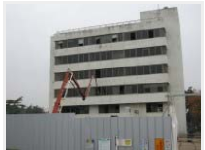
KEK's Building 2 under renovation.
