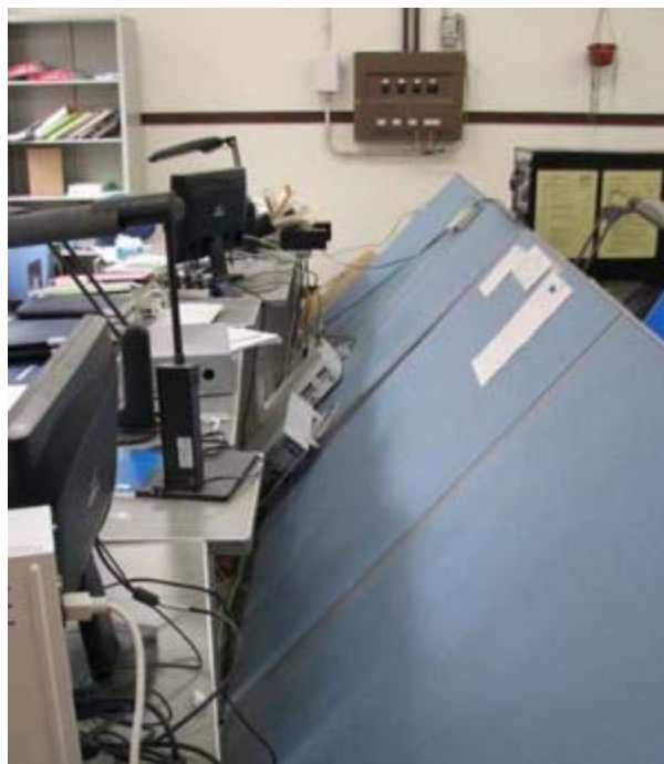
Fallen partitions at Tohoku lab, just after the 11 March earthquake.
