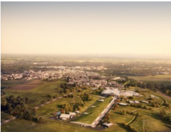
Experience gained at the European Spallation Source currently under construction in Sweden was fed into the Project Implementation Plan. Image: ESS
