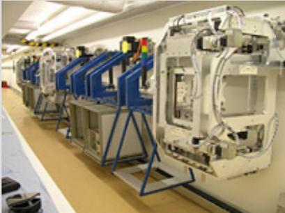
A three-car LiCAS RTRS system in the first stages of installation in DESY's 'red-green' tunnel.
