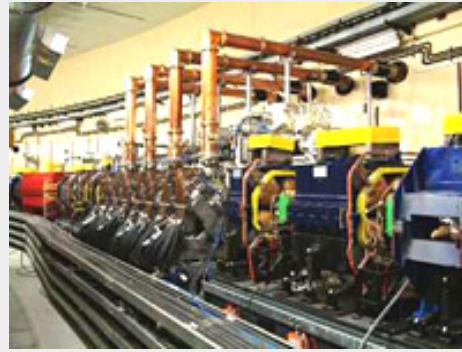
Indus-II Accelerator at Raja Rammana Center of Advanced Technologies (In View RF Cavities).
