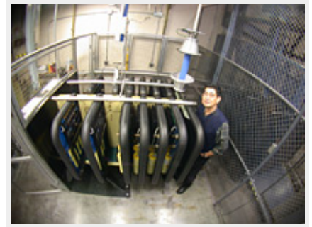
The Marx Modulator Test Facility at SLAC.
