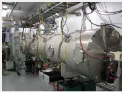
The SNS' cryomodule 19 in the test stand just after commissioning and fully qualifying it for the accelerator.
