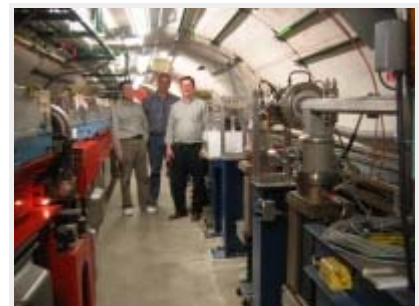
Yulin Li (Cornell), Robert Holtzapfle (Alfred University) and Mark Palmer (Cornell) in the ring during last week's downtime when modifications were made to transform CESR into CEsR-TA.
