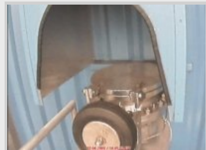
Helium escapes through a safety flap of the crash test cryomodule's safety valve which protects the 2K cavity helium volume inside the cryomodule against too much pressure. Click here to download the video (3.5 MB).
