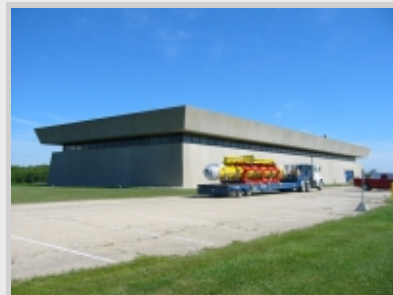
The first cryomodule on its way into the NML hall at Fermilab...
