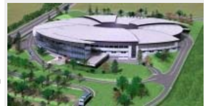
The ALBA Light Source Facility, under construction near Barcelona
