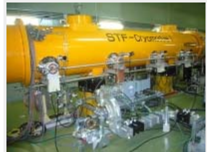
High-power tests of the first installed cavity in July 2008
