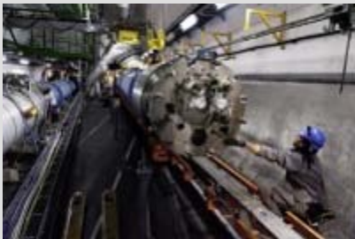
Transport of a LHC magnet to the surface in order to be repaired. Credit: CERN
