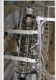
Cavity electro-polishing system installation at DESY.
