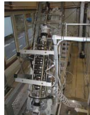
Cavity electro-polishing system installation at DESY...
