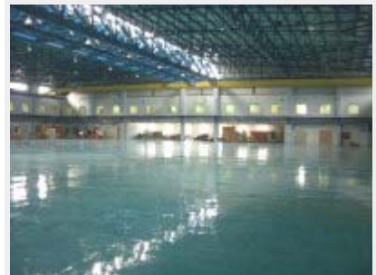
The large SESAME building, 75 metres by 75 metres, built by the Jordanian government
