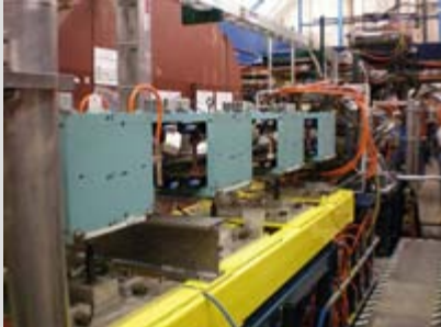
Magnets in blue-green boxes hug the beam pipe at CEsrTA. This setup tests how magnetic fields affect electron clouds.
