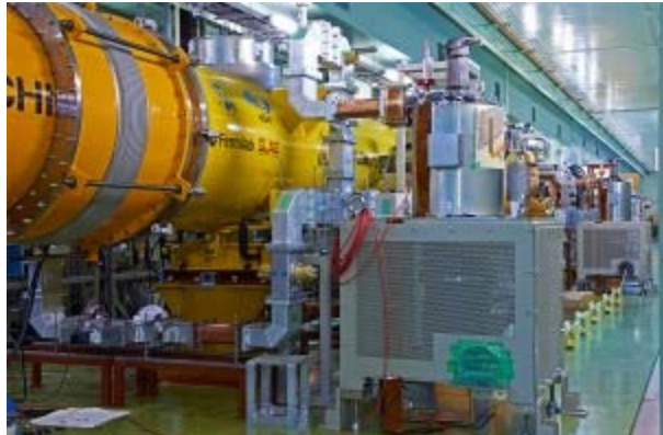
Hardware equipment for DRFS has been installed and being tested at KEK's STF. Image: Nobu Toge
