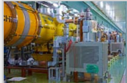
Hardware equipment for DRFS has been installed and being tested at KEK's STF. Image: Nobu Toge
